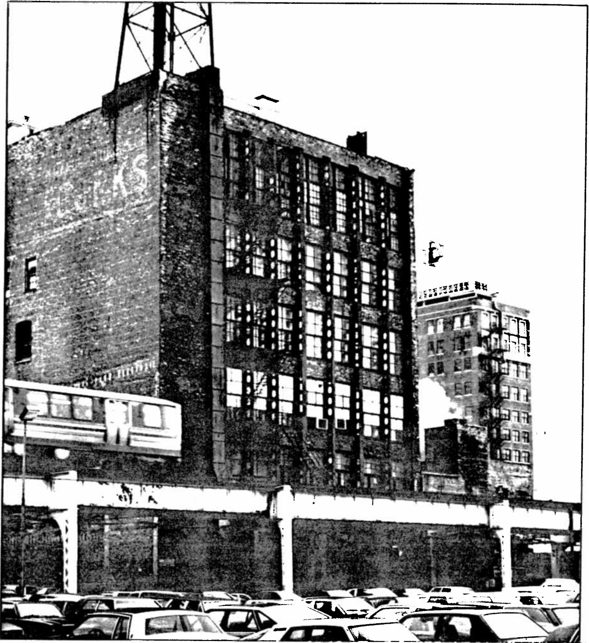
On the alley elevation, perforated cast iron braces the back wall in order to open it up as much as possible for natural light on the interior. ( Timothy Barton, photographer )
